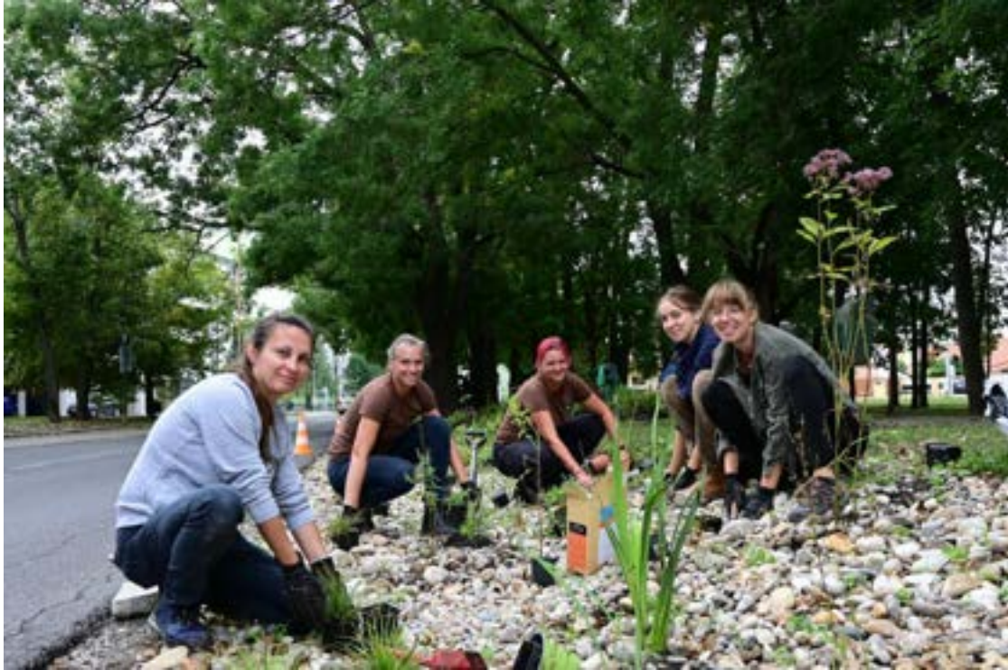
Fig. 4.20.4. The completed rain garden and the builders.
