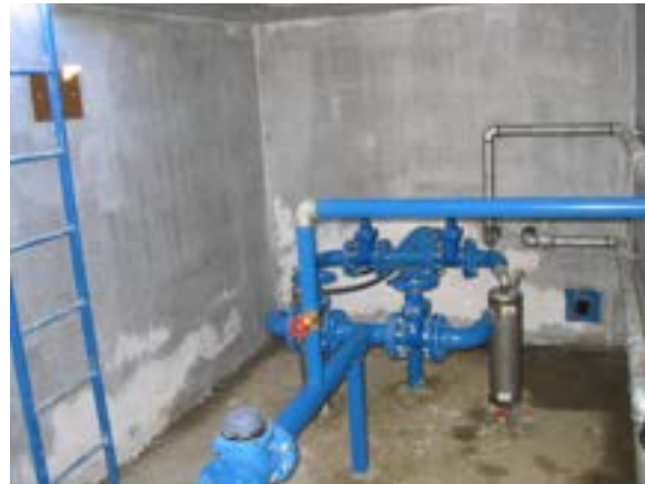
Fig. 4.15.3. Groundwater well providing heat.
