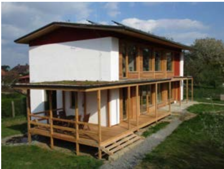
Fig. 4.9.4. Passive house ready for living
