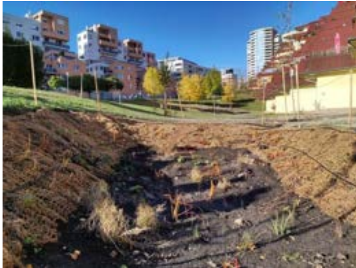
Fig. 4.19.3. The basin for the rain garden.
