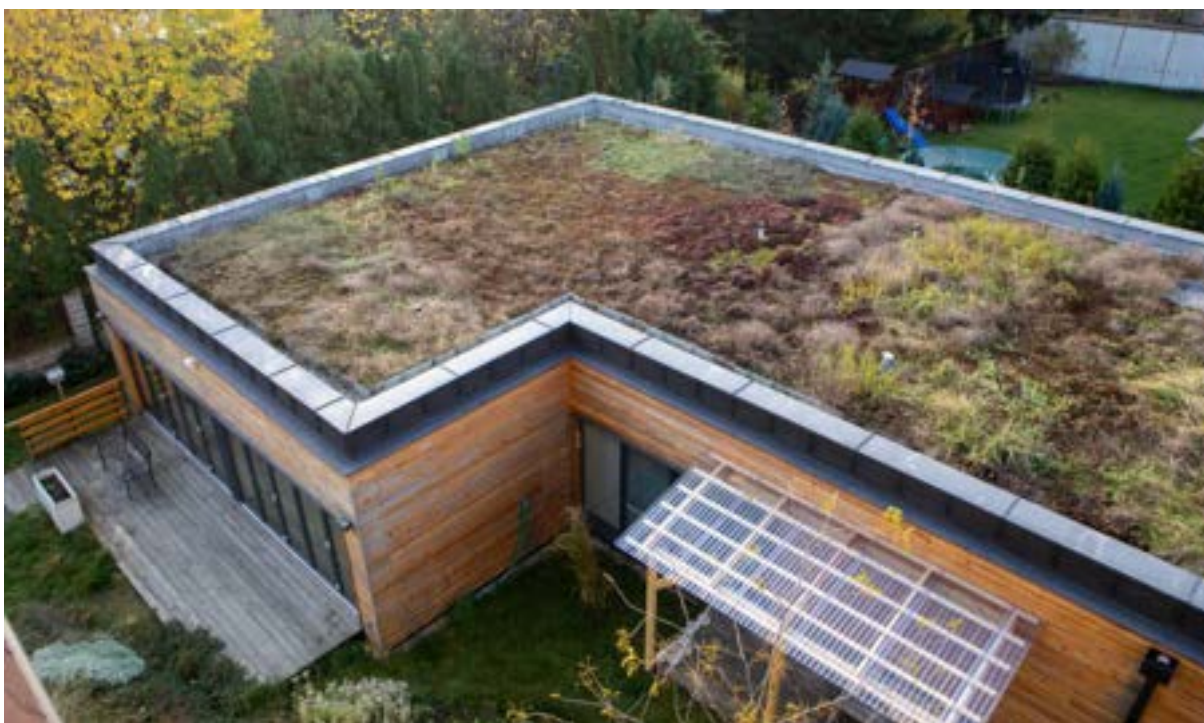
Fig. 4.7.3. Extensive green roof.
