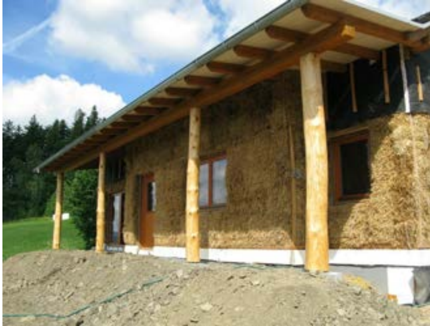
Fig. 4.9.3. Traditional design but innovative and green building method.
