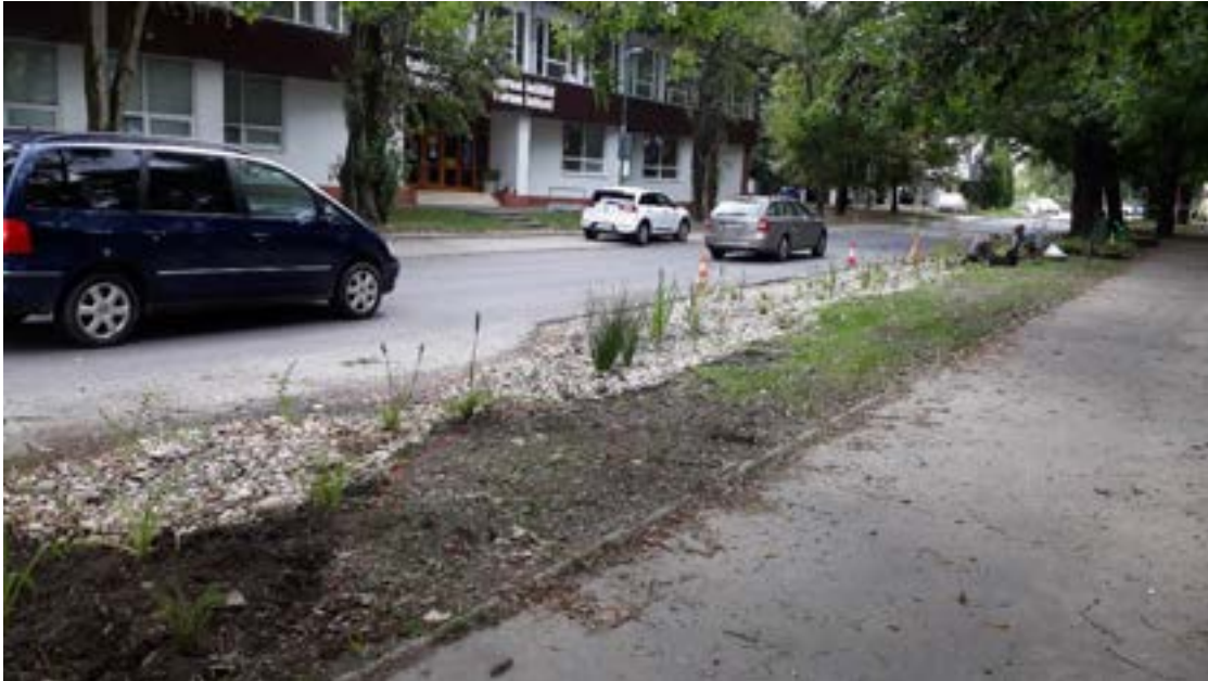
Fig. 4.20.5. The complete rain garden.
